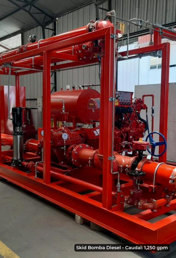
Skid Bomba Diesel - Caudal: 1,250 gpm
